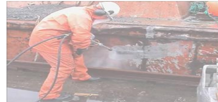
Sand/Water jetting: L_{pA} = 90 dB
