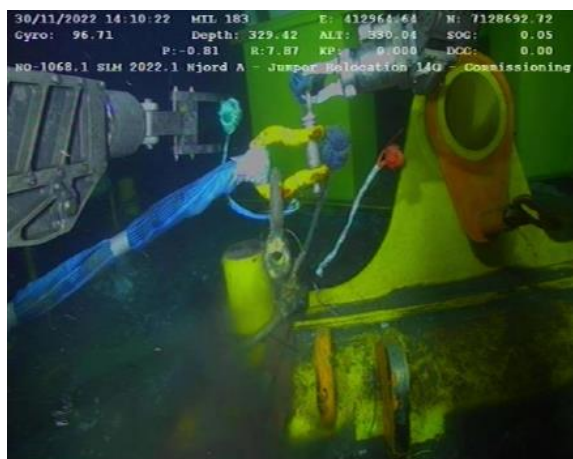
Figur 6-155 Hold back rigging demonteres fra jumper 14C, 1. ende
