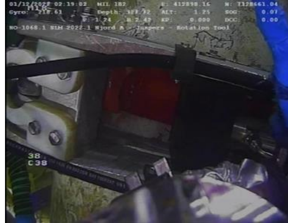
Figure 6-133 Jumper 14B Well End Rotation Attempt using Rotation Tool
