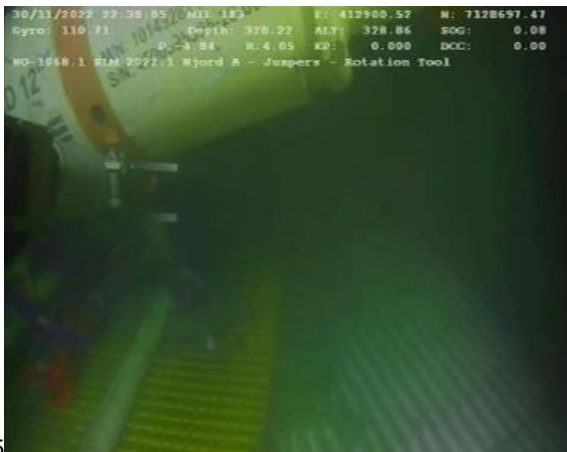
Figure 6-128 Jumper 14C Well End Rotation Attempt using Rotation Tool
