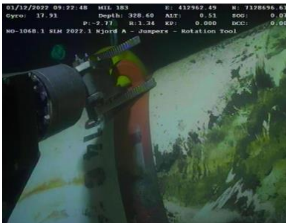
Figure 6-142 Jumper 14C SMS-N End Rotation Attempt using Rig Master
