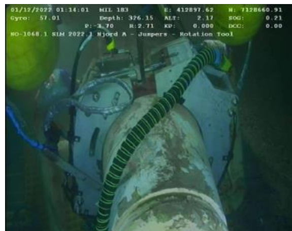
Figure 6-131 Jumper 14B Well End Rotation Attempt using Rotation Tool
