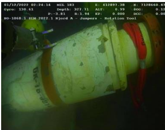
Figure 6-134 Jumper 14B Well End Rotation Attempt using Rig Master
