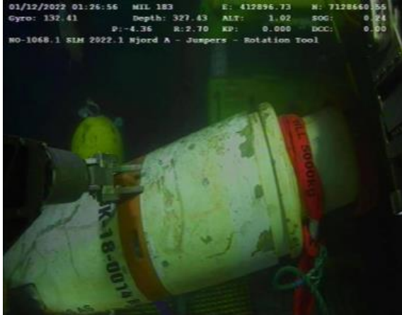
Figure 6-132 Jumper 14B Well End Rotation Attempt using Manipulator
