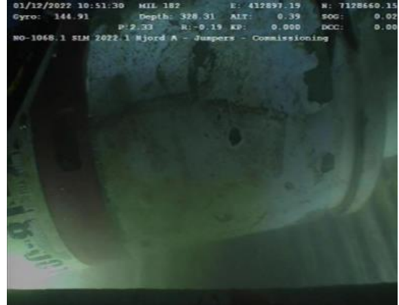
Figure 6-145 Jumper 14C SMS-N End Rotation Attempt using Manip
