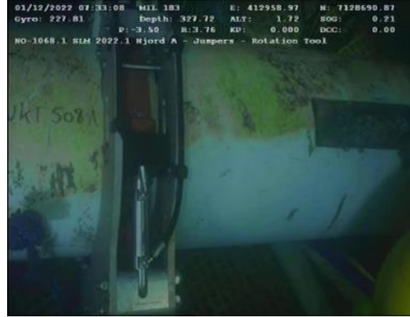
Figure 6-139 Jumper 14B SMS-M Rotation Attempt using Rotation Tool
