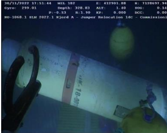
Figure 6-126 As-Found Jumper 14C Well End
