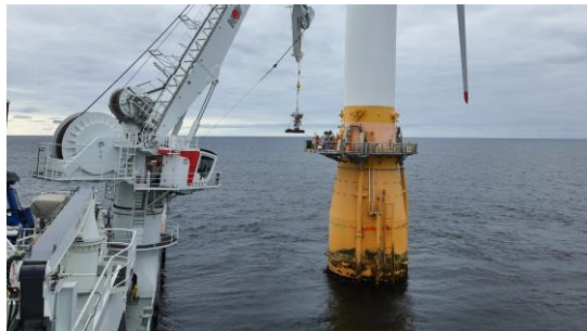
Crane service to unmanned offshore floating wind turbines
