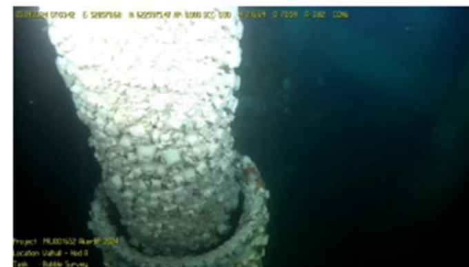
Picture 15: Conductor 8 (69m) - No leak observed
